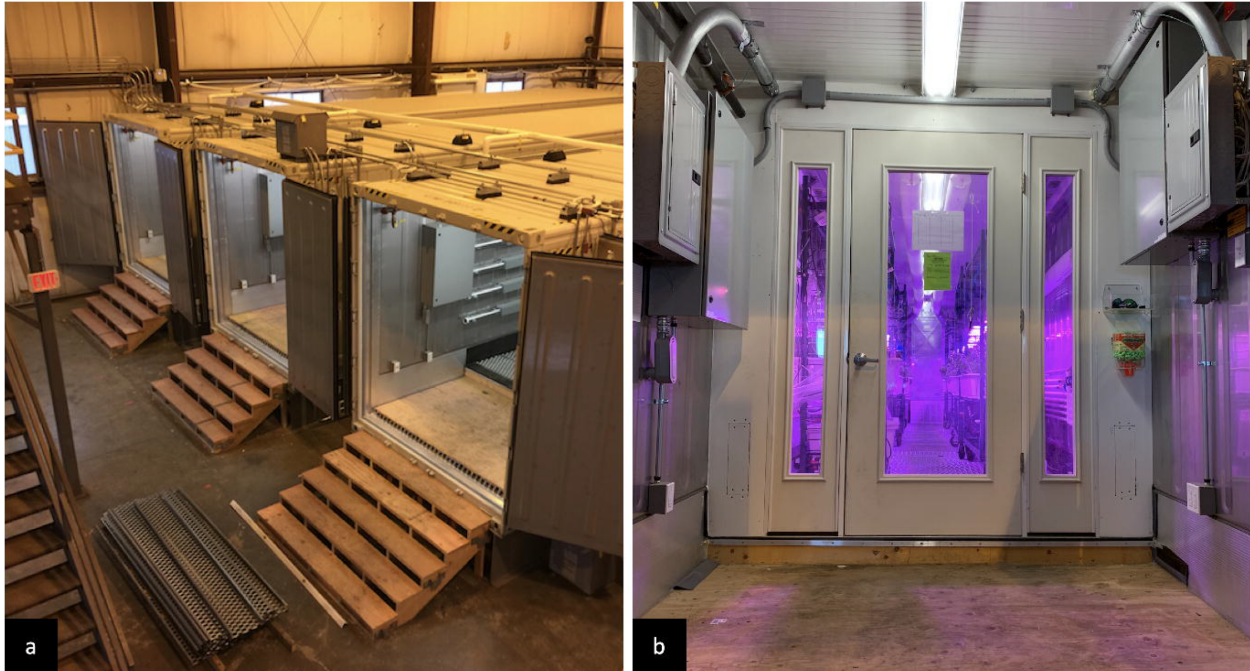
Figure 5: The MIT expansion facility under development. (a): Four containers being converted to large-scale Food Servers (b): The entrance to the next generation of MIT OpenAg Food Servers.
